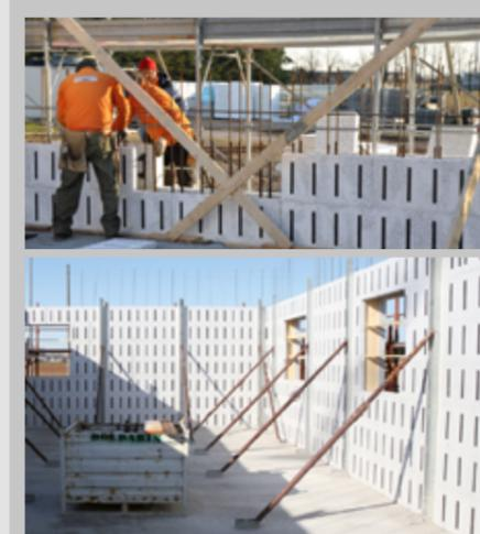
Proceed up to the envisaged height and fix the alignment and plumb line measuring system to the Climablock.
