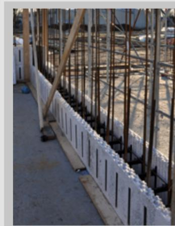
Position the reinforcement which, as a final result, will form a mesh consisting of horizontal and vertical rods similar to electro-welded mesh.
