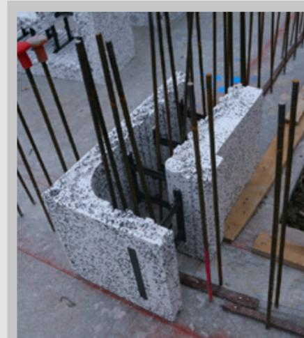
Start the first section starting from the corners and continue with the installation of the linear blocks.
