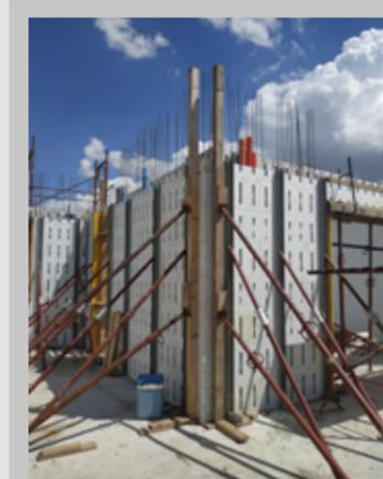
Adjust the alignment and plumb line measuring just before casting. Cast using S4 concrete (thixotropic type, max aggregate granulometry 20 mm).
