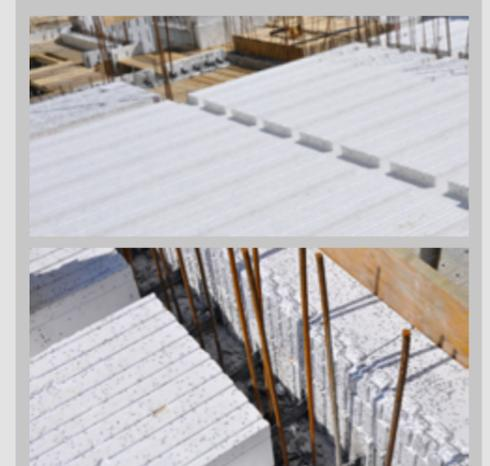
When creating the slab, the continuity of the external insulation is not interrupted, thus avoiding thermal bridges; moreover, the edge of the slab has already been made.
