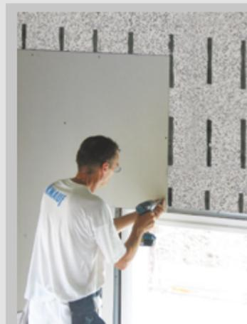
The brackets of the block allow fastening of the internal finishing cladding without creating the dedicated structure.
